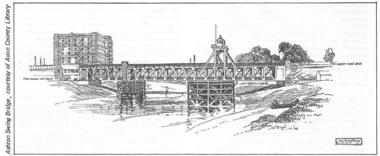
copper pipes (with steel cables laid 50 yards upstream and downstream to protect them from vessels dragging their anchors) to the cabin on top of the bridge where the hydraulic machinery was located:-
